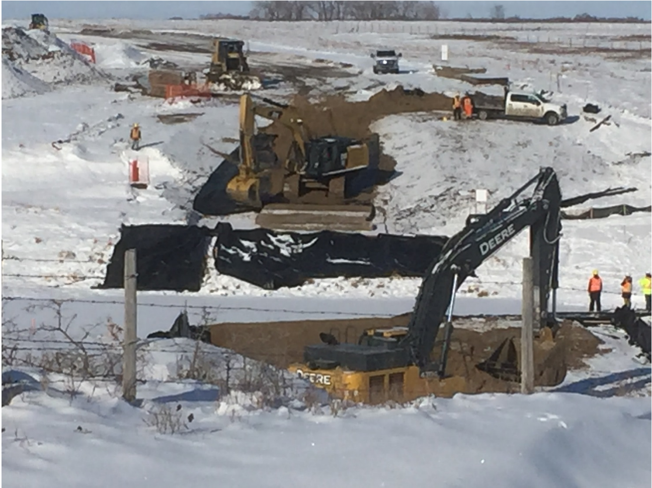
HIGH HILL CREEK BEFORE BRIDGE INSTALL
